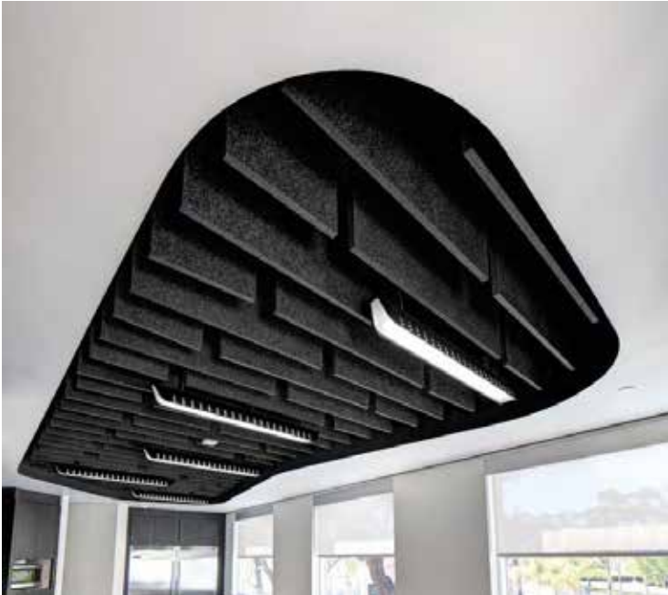
An example of acoustic ceiling baffles being considered for the SUB. Ceiling baffles will provide much needed acoustic control in the north / south corridors.
