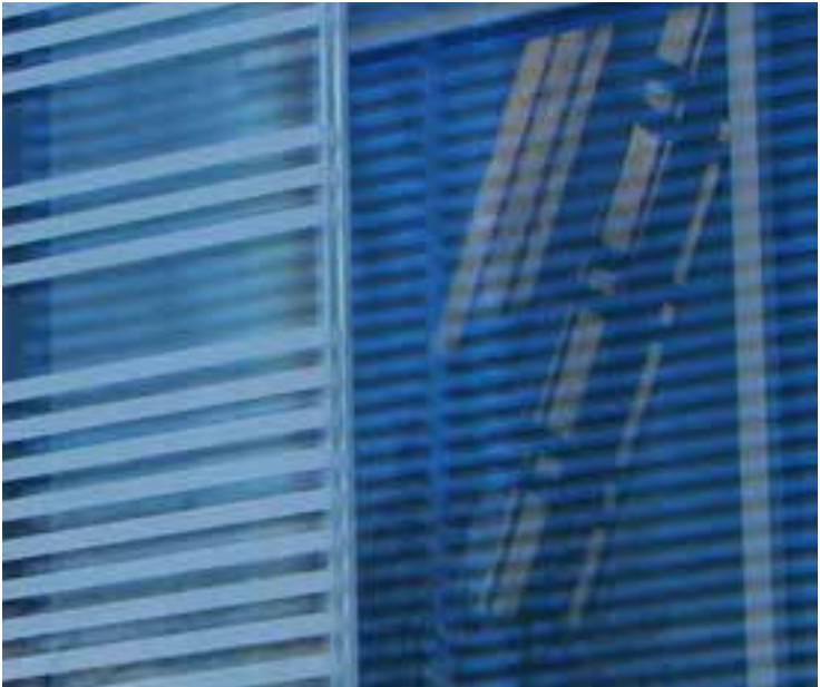
Glass: Glass will be used for windows, as well as vertical fin elements that relate to the SFU architectural language. Glass also provides transparency to make the building open and welcoming. Exterior vertical fins act as shading devices and will have a translucent interlayer to reduce glare inside the building.
